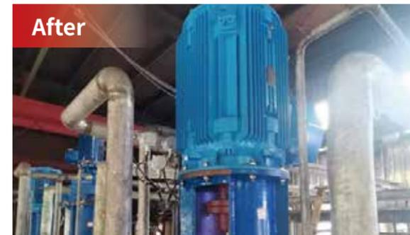
The original system has problems such as transmission gear box bearing oil leakage, high energy consumption etc. Permanent magnet direct drive retrofit completely eliminates the transmission gear box, lower down downtime and use a supporting frequency converter to control the motor operation, so as to achieve energy saving rate of 32.5%.
